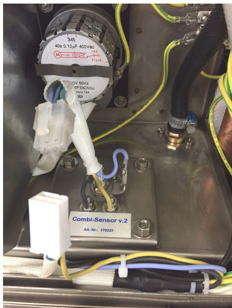
Pull off the sensor plug (6-pin)
